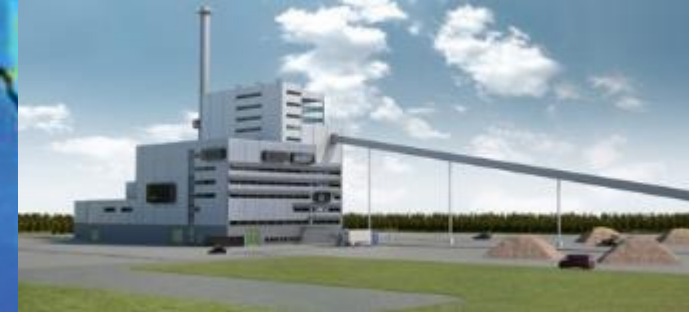
Visit at the Örtofta combined biomass heat and power plant.
